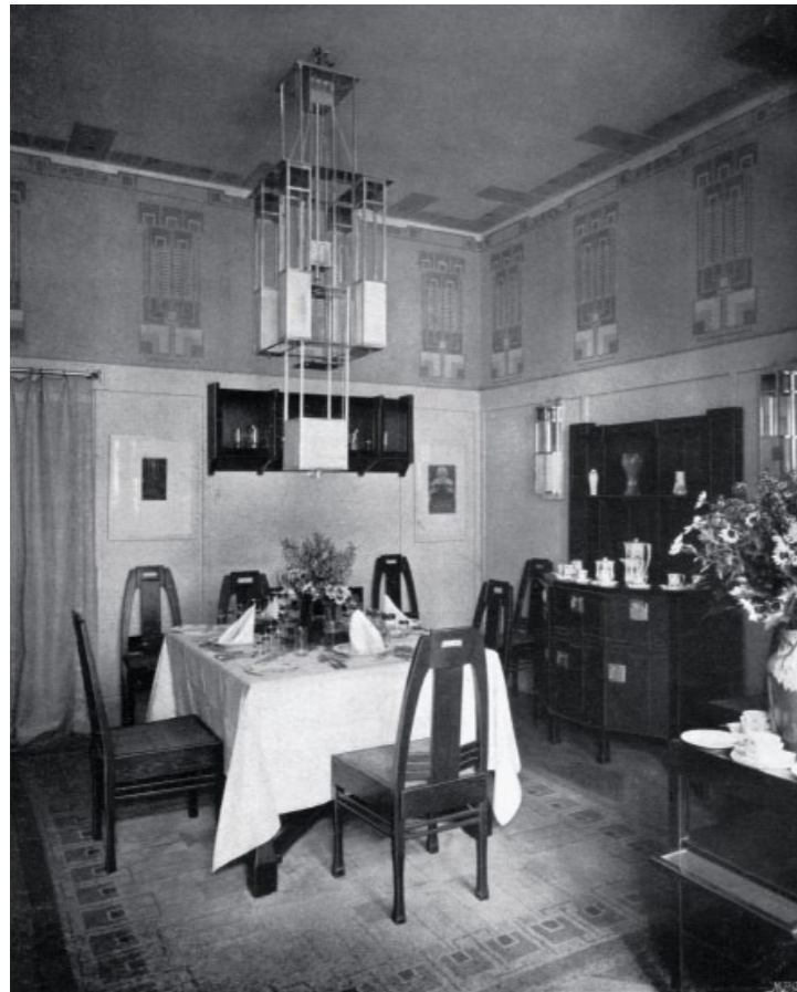
Dining room installation at the Wertheim department store, 1902
